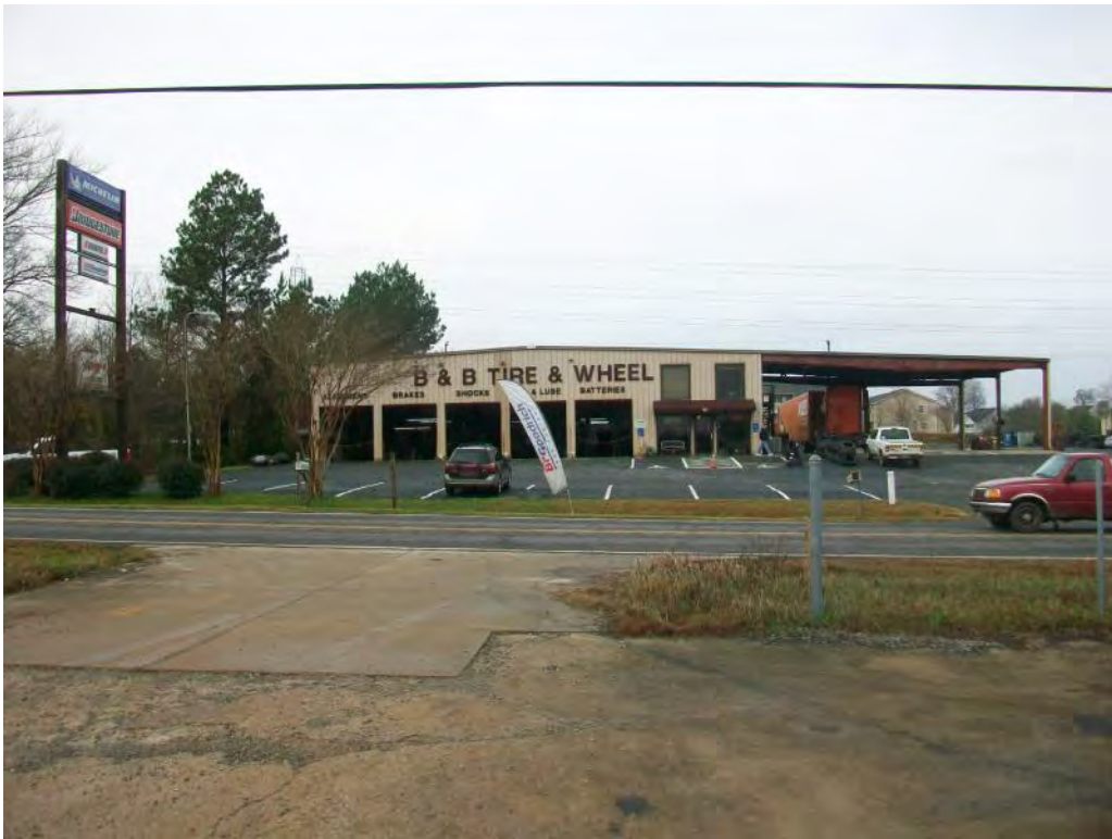
Photograph 7 – View of B&B Tire and Wheel located adjacent to Riverview Road.
